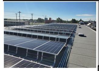
Construction of the solar array on the THRC is now complete. It is estimated that significant operation savings will be delivered through 136 x 400 watt panels. The project would not have been achieved without significant support from the Municipal Climate Change Action Centre (MCCAC) and Municipal Sustainability Initiative (MSI) funds.
