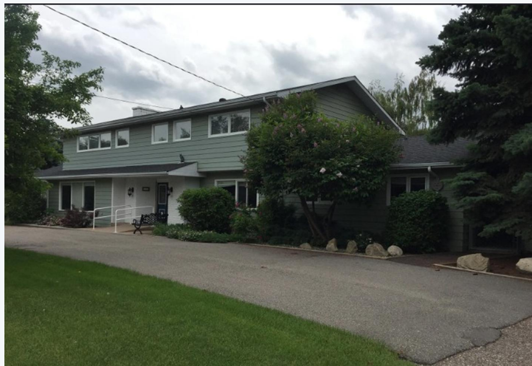
EXISTING HOME CARE BUILDING
