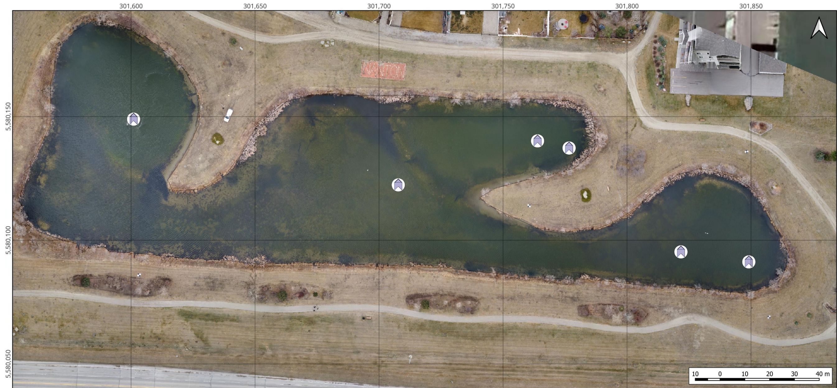
Figure 11 Westview Meadows Stormwater Pond sediment sample locations
