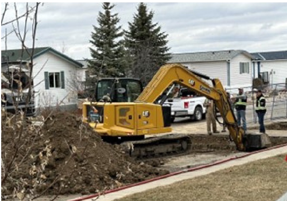
29 Ave Waterline Repair
