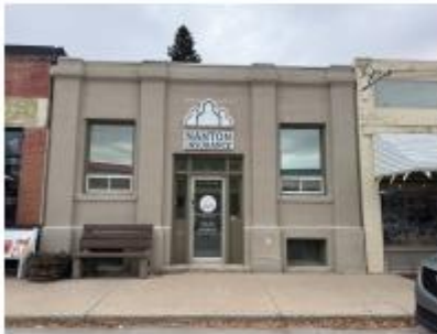
Nanton Telephone Exchange - 2118 20 Street (1918)
