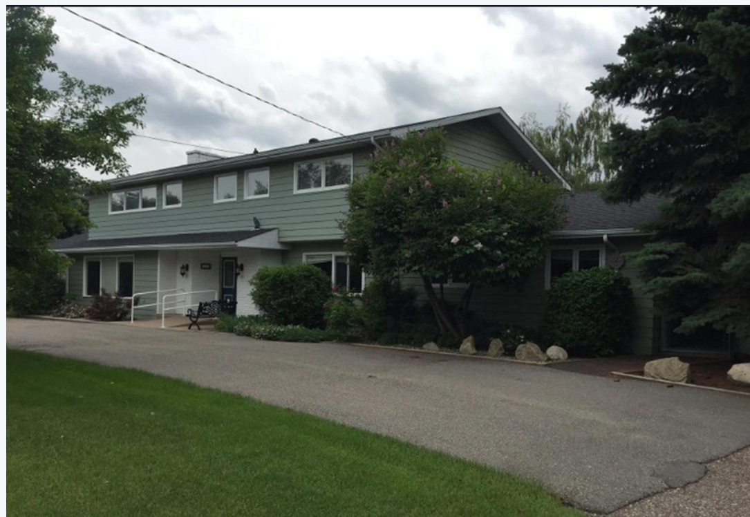
EXISTING HOME CARE BUILDING
